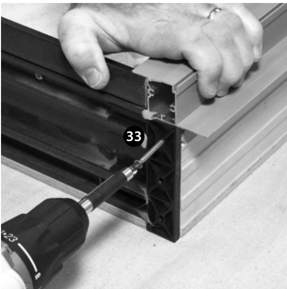
Join Together and Fasten Through the Bracket
