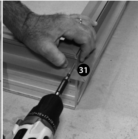
First Fastener (31) at Edge Hole
