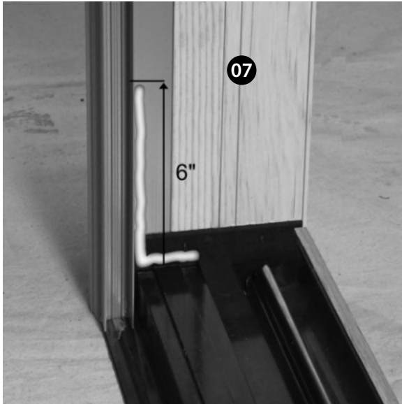
Apply Sealant 6" Up Jamb Recess
