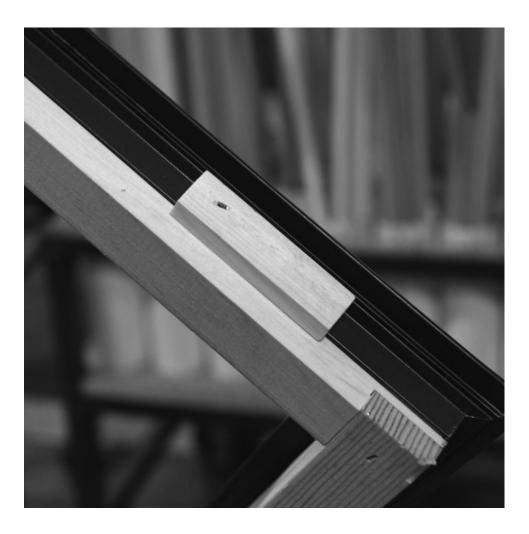
Sun Casement windows have a Shipping Block installed on the bottom of the operating sash to prevent damage to the sash and operating hardware while the window is being transported. This Shipping Block must be removed during the installation process. Failure to remove the Shipping Block will result in poor performance of the window and possibly the inability to open the sash.
