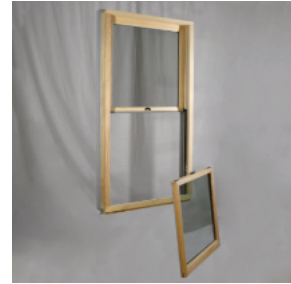
8. The bottom sash is now removed from the window.
