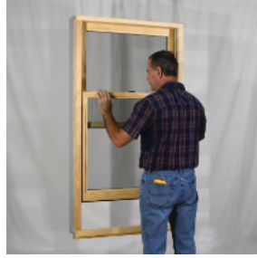
2. Raise the bottom sash approximately 6 inches.
