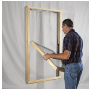
14. Lift the other side of the sash until it is clear from the other Sash Pivot Shoe.
