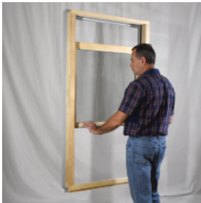
9. Lower the top sash approximately 6 inches.
