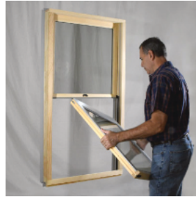
7. Lift the other side of the sash until it is clear from the other Sash Pivot Shoe.
