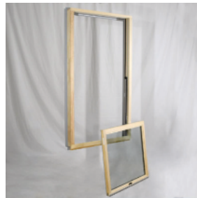
15. The top sash is now removed from the window.
