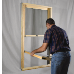
6. Lift up one edge of the sash until the bottom of the sash is clear from the Sash Pivot Shoe in the Side Jamb Track.
