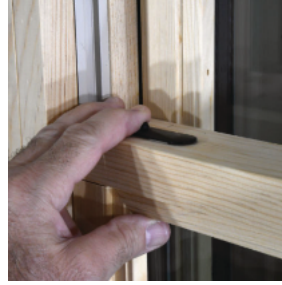
3. Grip the Sash Tilt Latches at both sides of the Checkrail and slide them towards the center of the sash to disengage the latches from the side Jamb Tracks.
