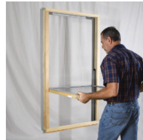
12. Tilt the sash until it is approximately 90° perpendicular.
